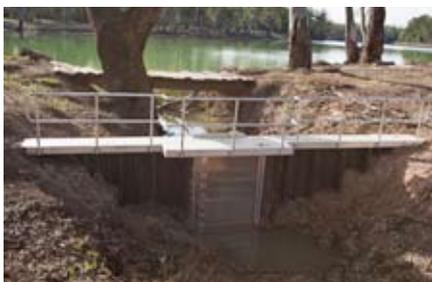
Above: A Plastipile environmental regulator, similar to what will be built at Baggs Bridge and Jennings Bridge. Photo: Mallee CMA.
